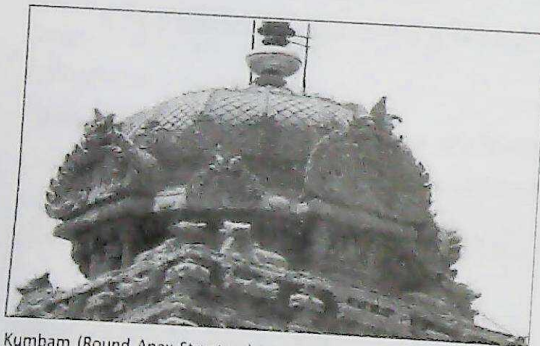
Kumbham (Round Apex Structure) is carved from a single granite rock. It weighs approx. 80 tons and sits on top of the temple tower. The Vimanam (Temple tower) is 66 meters (216 feet high). How did workers 1,000 years ago manage to lift an 80-ton carved stone this high... Without any cranes or lifting machines, still remains a mystery.
