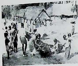
Digging canal in the Harijan Colony, Kovur
